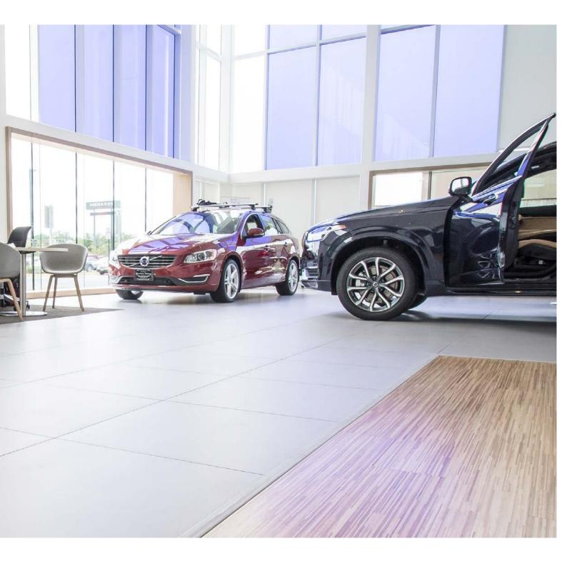
Large format tiles you can drive car over? Sure. Mosa offers measurable performance standards that provide extra insurance to specifiers and their retail clients in areas of breaking strength and modulus of rupture. These same characteristics also make Mosa the choice of architects to prevent failures due to the heavy, dynamic loads and sustained vibration inherent in retail environments such as auto dealerships.
